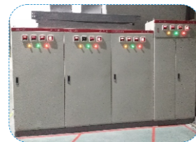
低压配电 Low-voltage Distribution
