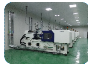
车间管路 Workshop Pipeline
