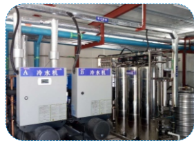
工艺冷冻水 Processing Chilling Water
